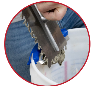
Scrape to remove excess material
