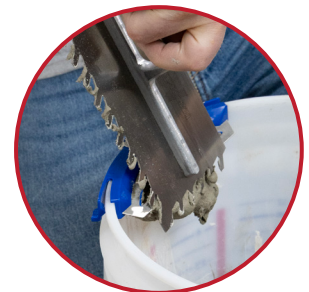
Scrape to remove excess material
