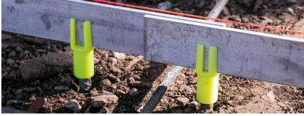
**Bypass Support** Chairs can hold two rails side-by-side to bypass one rail to another
