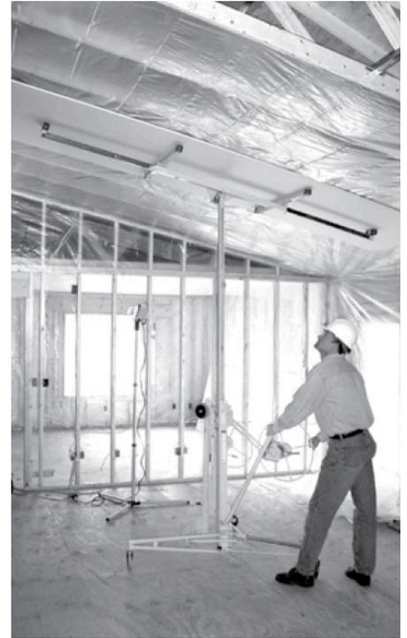
**1.** To Load: Set the backstop on the tripod base to hold the unit in position. Extend the cradle outriggers to properly support the drywall, tilt the cradle, and swing out the cross arm support hooks. Load the MARSHALLTOWN Drywall Lift from the front as shown with the face paper of the drywall contacting the cradle.
